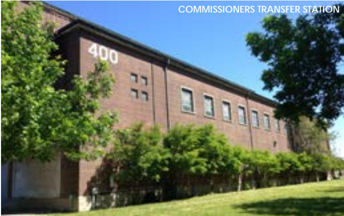
COMMISSIONERS TRANSFER STATION
